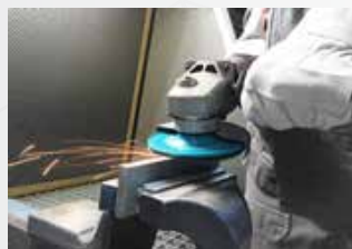
Weld seam preparation
