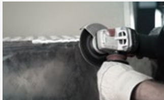
Removing welded seams
